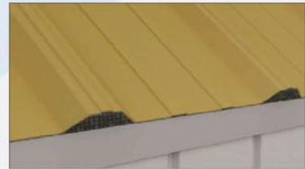
Step 3: Place the roof panel over pre-cut closure configuration for a snug fit. Attach panel over closure with the proper fasteners.
